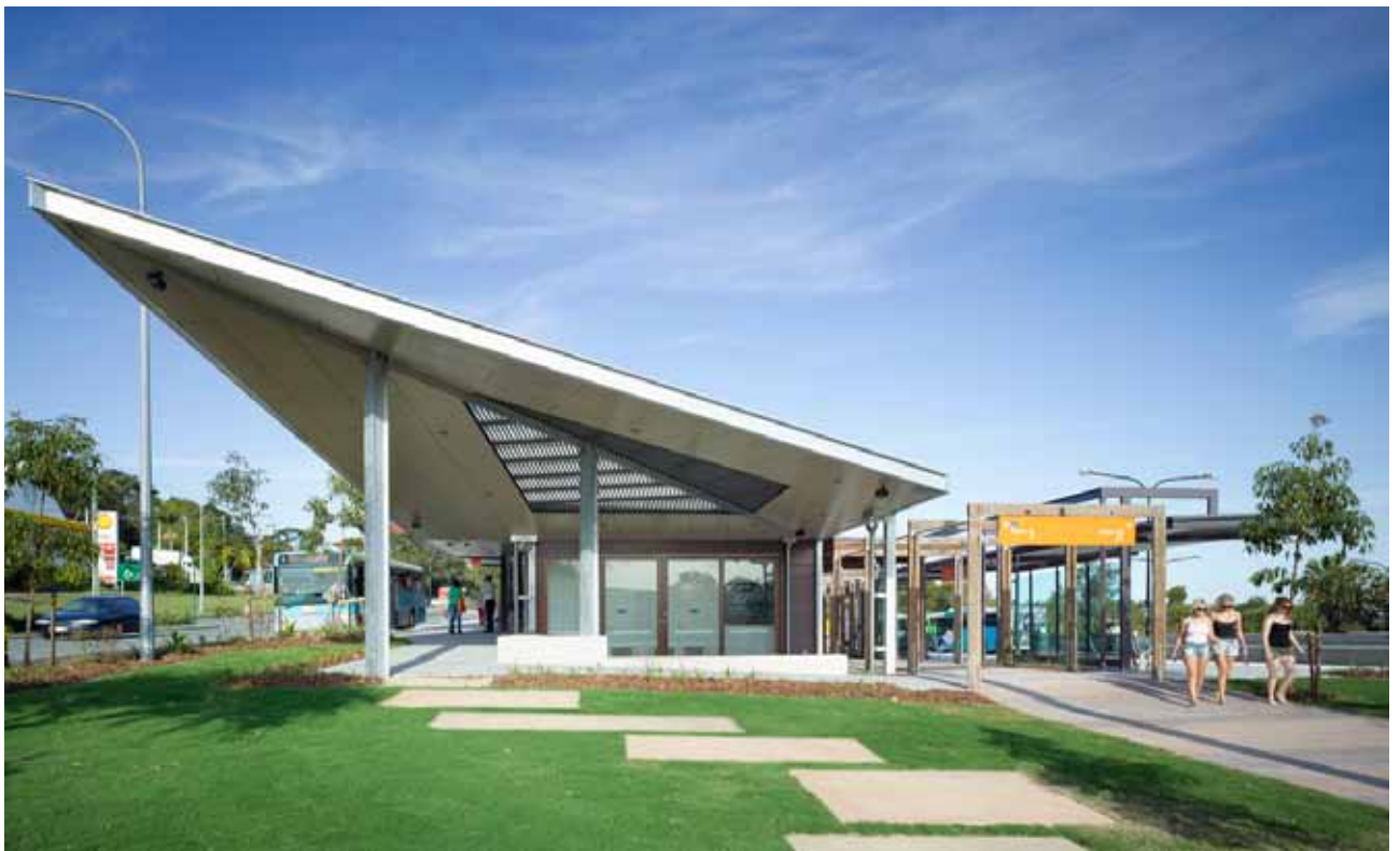
Multi award winning Noosa Junction Station, Sunshine Coast, Queensland
