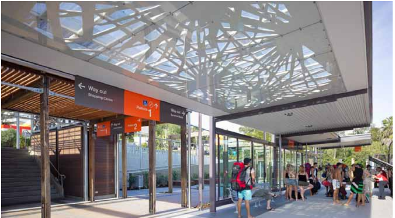
Multi award winning Noosa Junction Station, Sunshine Coast, Queensland
